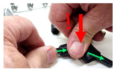
After getting wire through boot, pull at least 6 inches through, leaving room to strip and then terminate the end. Considerable force is required to do this. The dielectric grease wipes off easily.
